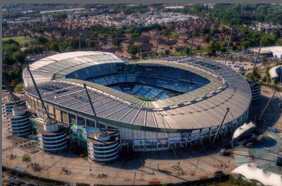
Etihad Stadium (Manchester City) - United Kingdom
